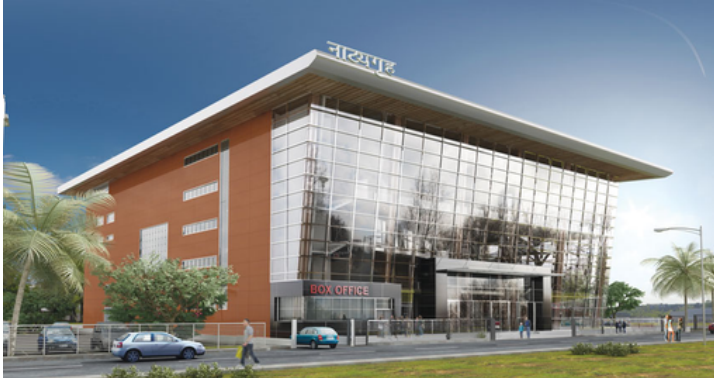
Community Cum Convention Center Multi-storey building
